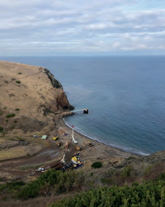
Preconstruction view of Scorpion Anchorage pier site
