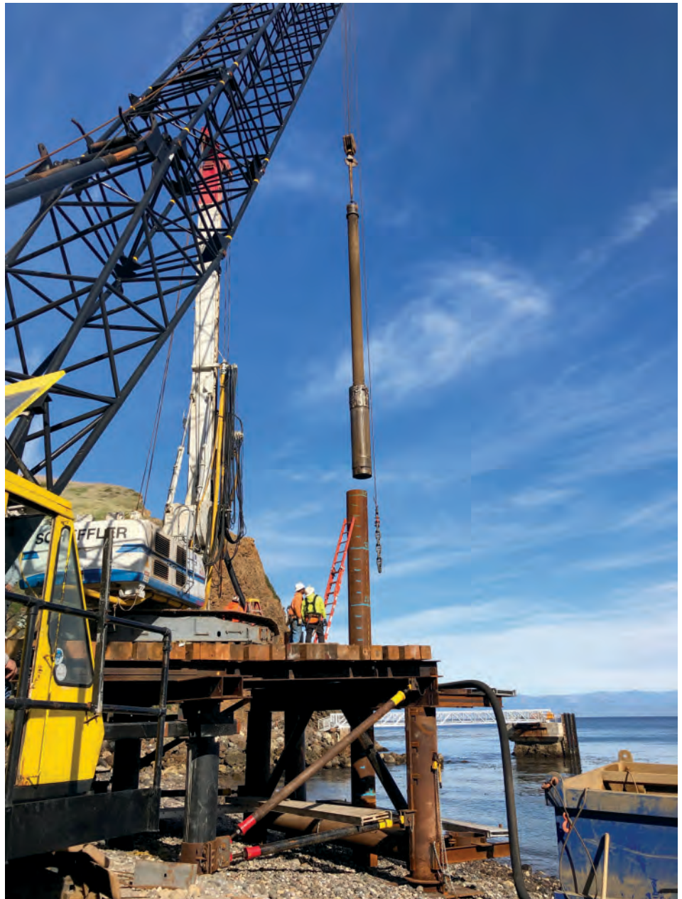
Inserting down-hole hammer into casing at shoreline
