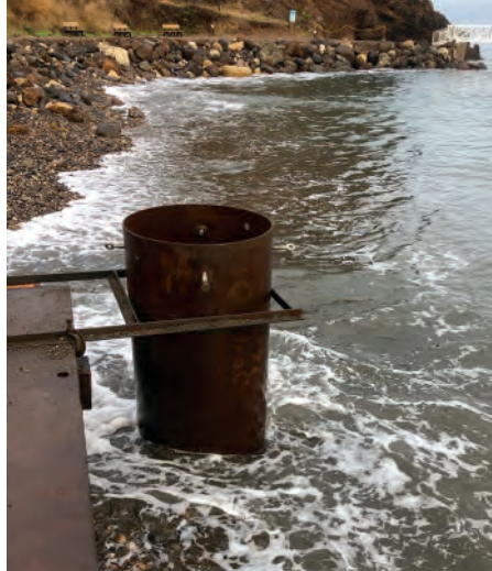
Pile drilling guide near shoreline
